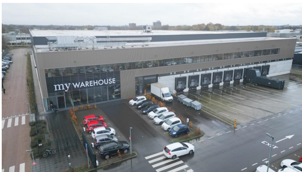
The new distribution centre in Den Bosch is expected to receive the BREEAM Excellent in-Use certification by the end of 2024.
